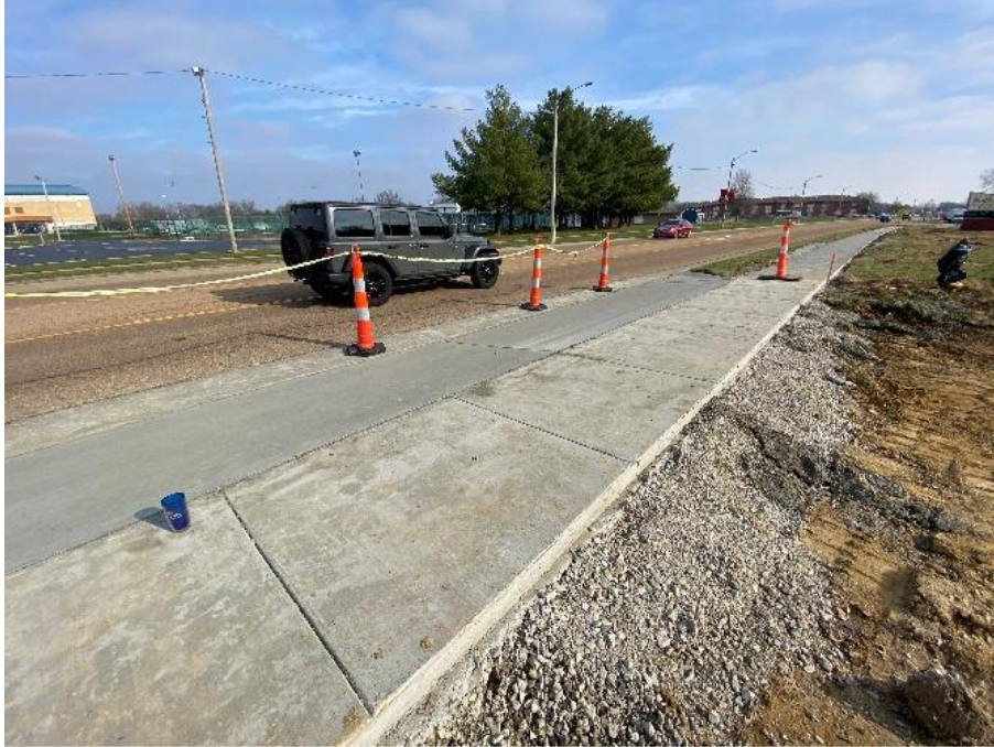
New sidewalk along Highway 50
