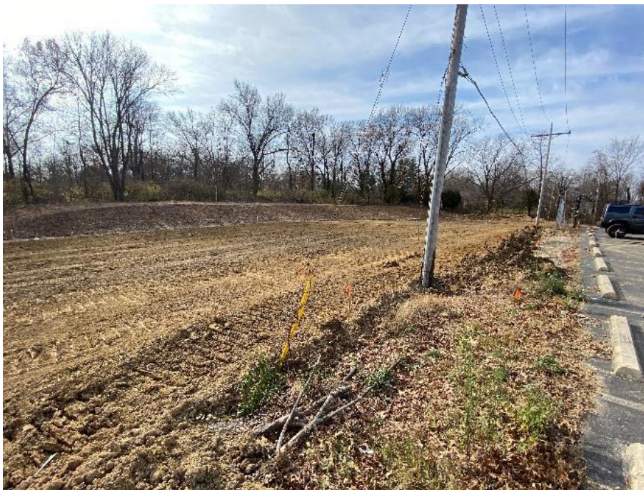
Excavation, drainage, and parking lot expansion preparation
