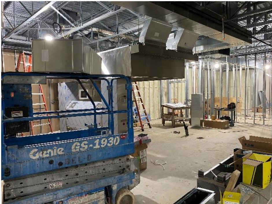
Kitchen ducting, interior walls, and cooler/freezer preparation
