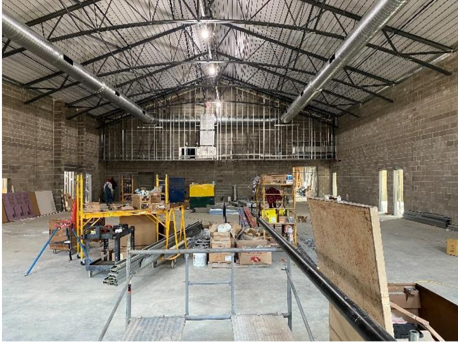
Fellowship Hall (facing east)
